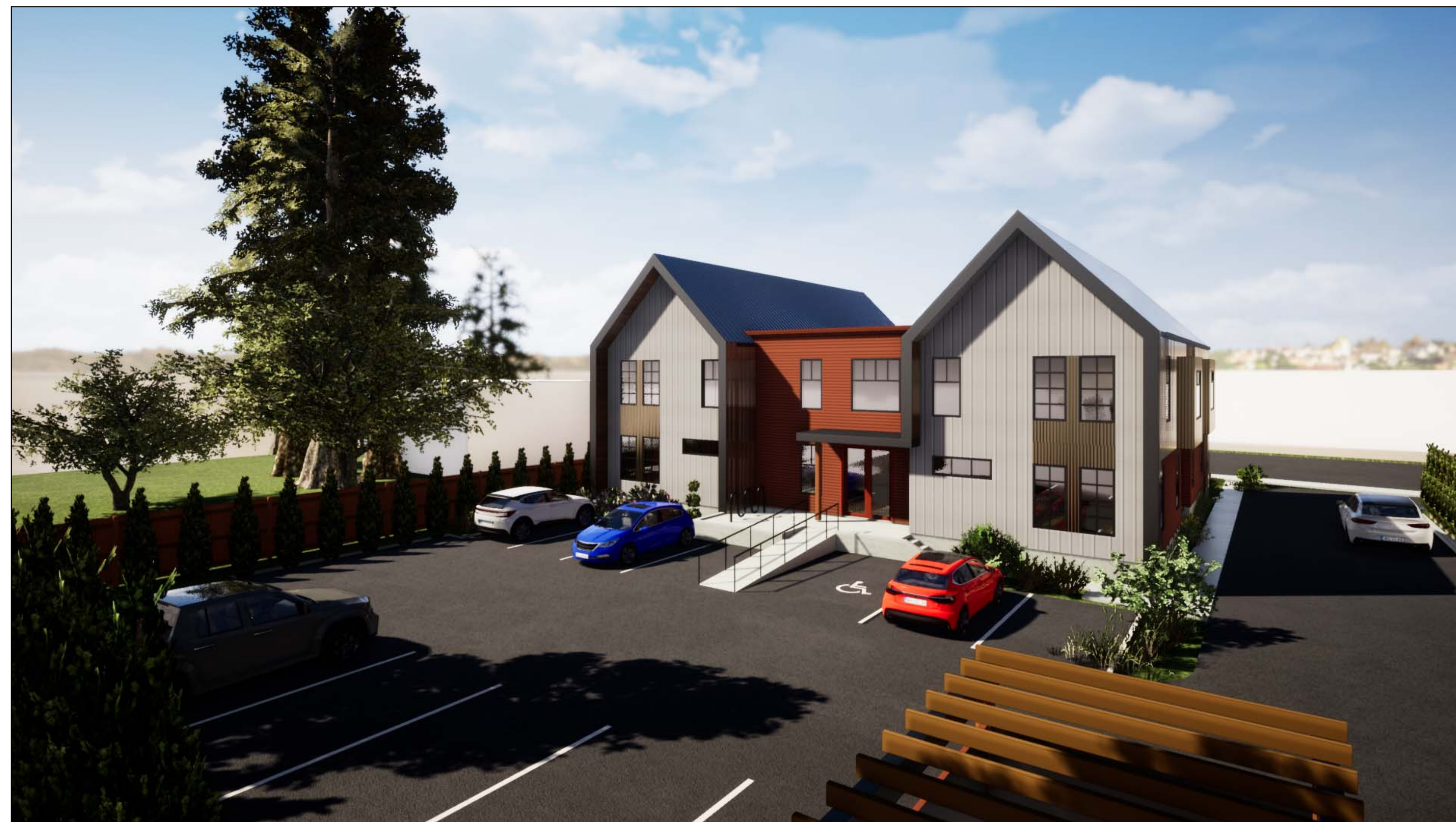
VIEW FROM SOUTH-EAST CORNER
